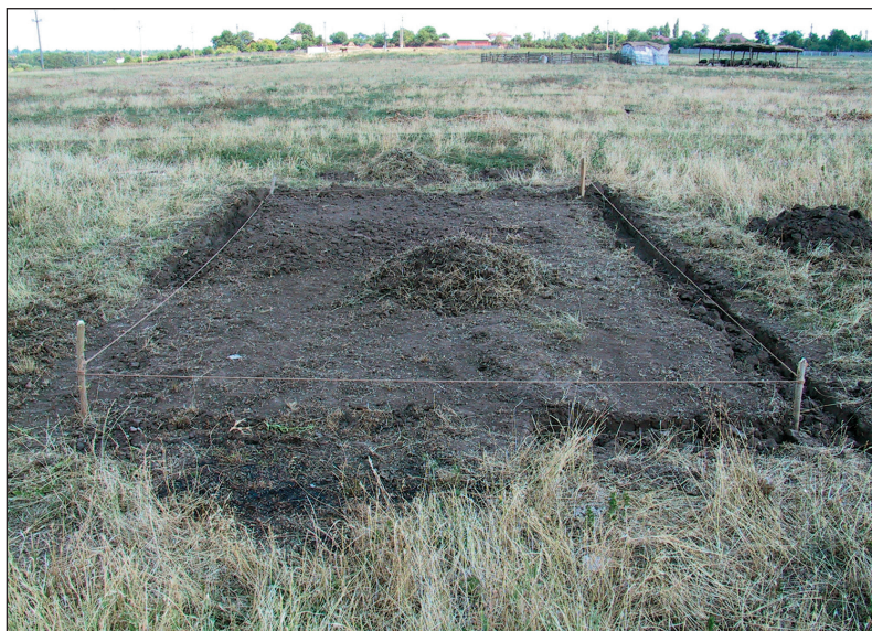
Fig. 4. Foundation ditches for a wattle and daub house, Vadastra 2003.
