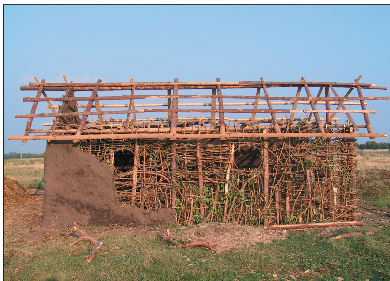
Fig. 5. The plaited structure of walls. Vadastra 2005.
