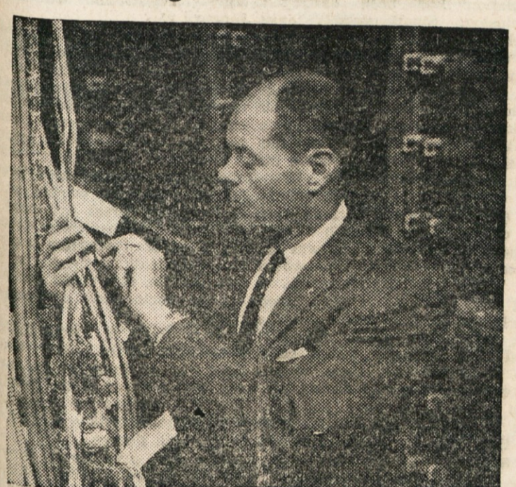
OHIO BELL PRESIDENT FREDERICK R. ECKLEY, who has announced the launching of a five-year, $680 million construction program to meet soaring demands for communications services, inspects new cable being connected to switching equipment at the site of one of the company's many expansion projects throughout Ohio.
