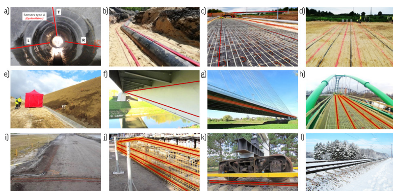
Figure 1: Example applications of distributed monolithic sensors to monitor various structures.
