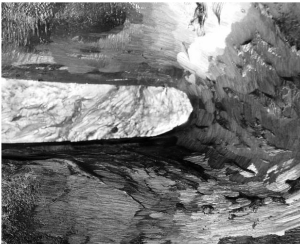
Figure 4: Crack surface with a repair-weld build up at the blade leading-edge attachment to the hub
