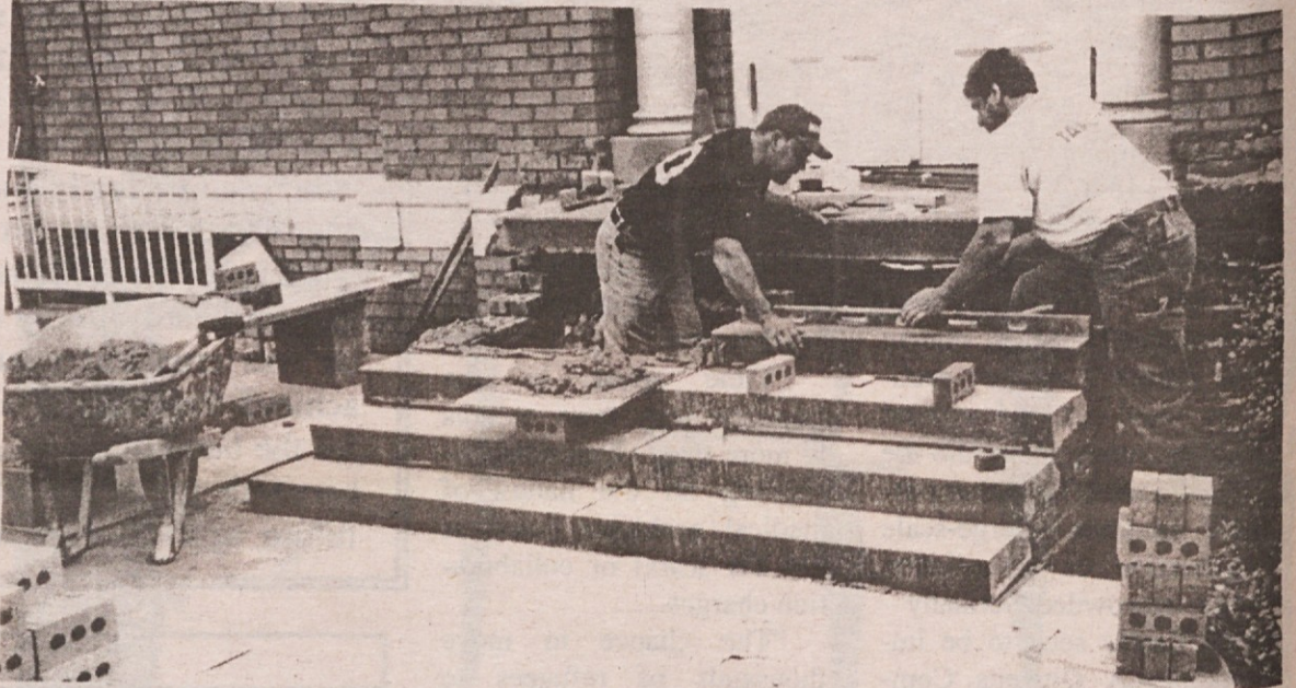
CORRECT AND LEVEL. – Sierpentowski (right-hand side) proprietor, Target Inc., and Tony Strnad (left), work together to ensure that one of many individual granite steps will be properly installed. They are completing work on the choir entrance steps.
