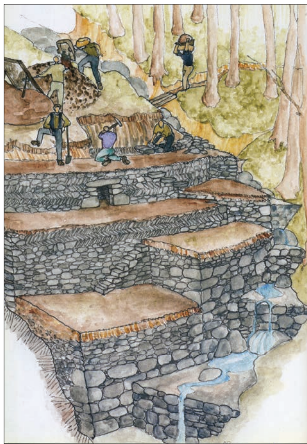
Figure 4: Final phase: walls 2-3 meters tall, terrace 3-5 meters. Various textures for the dry stone wall. Various types of access (stairs of exposed plates, walkable paths).
