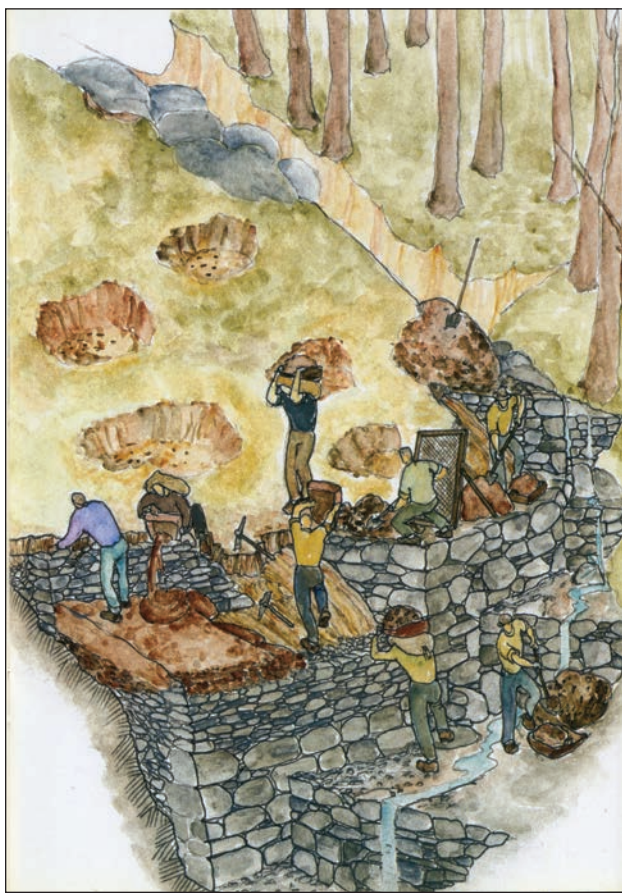
Figure 3: Trenching of the ground: Separation of the ground and stones (useful for the drainage). Completion of the river embankment.
