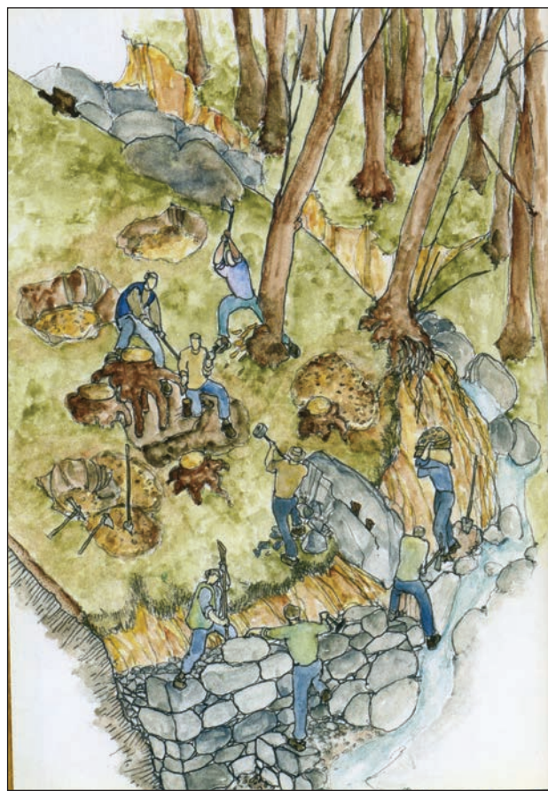
Figure 2: The settler or the owner decides to create a new small plot. A squad of daily workers-farmers begin to work. Starting phase: construction of embankment for the river and plot support.
