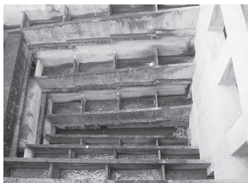
Slika 10: HE Mariborski otok - pogled na ribji prehod od zgoraj Fig. 10: Mariborski otok HPP - view of the fish passage from above
