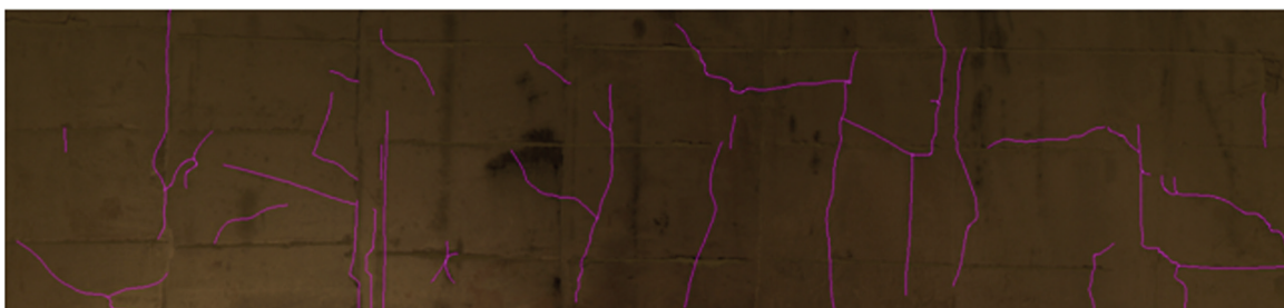
Figure 12: 2D mapping of fractures based on orthogonal photos.
