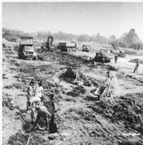
Sl. 13: Mengeš, gradbišče športne dvorane, ob prihodu na teren. Fig. 13: Mengeš, the building site of the sports hall, before the arrival of the archaeologists.
