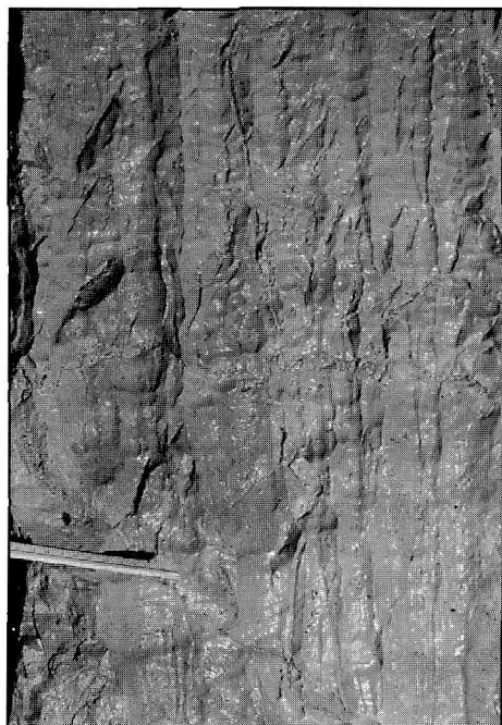
Fig. 8: The shafts wall shaped by trickling water
