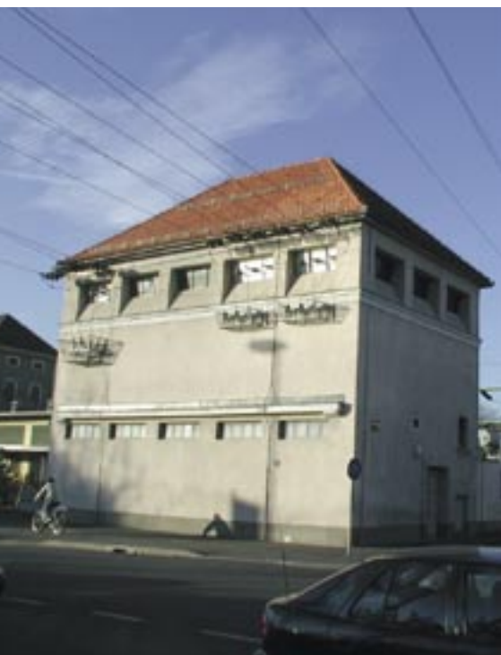
Obstoječa RTP 110/10 kV.
