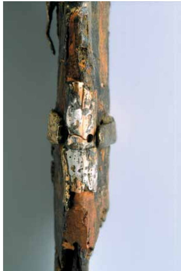
Fig. 6: The upper left solder-point of the guttering. Sl. 6: Spajkanje robnega okova na levi strani.
