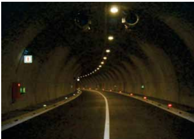
Figure 14. The final appearance of the tunnel when it was re-dedicated to a traffic 11. 11. 2009.
