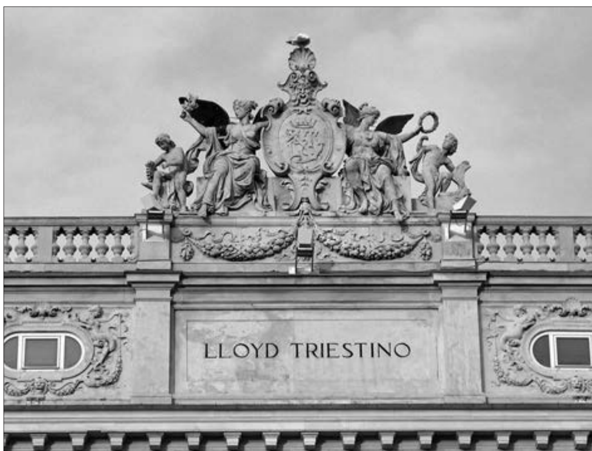
Okrasno čelo na Lloydovi palači v Trstu (Guido Linke, Freiburg [CC BY-SA 4.0 ( https://creativecommons.org/licenses/by-sa/4.0 )])
