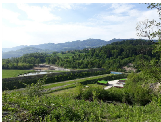
Figure 5: Remediated area above the mining area.
