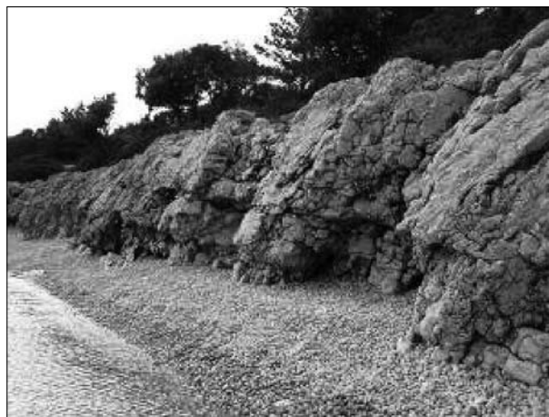
Fig. 9: Low coastal cliff at Martinšćica. Cliff is approximately 4 m high for scale (Photo: J. Mylroie).
