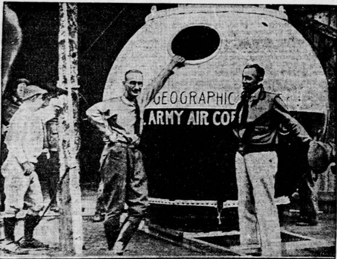
A. W. Stevens (na levi) in major William Kepner (na desni poleg gondole)
