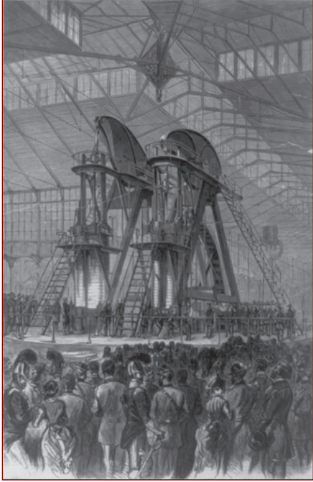
Figure 3: Illustration showing President Ulysses S. Grant and Emperor Dom Pedro II activating the Corliss steam engine at the opening of the Centennial Exhibition in Philadelphia. Based on a sketch by the artist Theo. R. Davis, the image captures the ceremonial moment that inaugurated the machinery hall and signaled the start of the international exposition. 66
