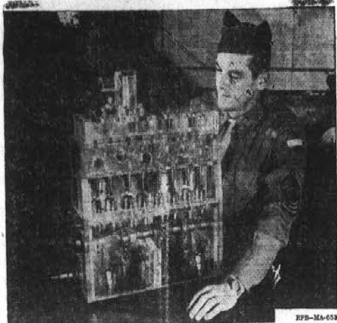
Visual clarity is obtained in this plastic model of a jeep engine built by M/Sgt. James Abbey of the Armored School, Fort Knox, Ky. Used in lectures in the Basic Engine Division of the school's Automotive Department, this transparent model enables the soldier-student to view the engine's interior parts while in motion.
