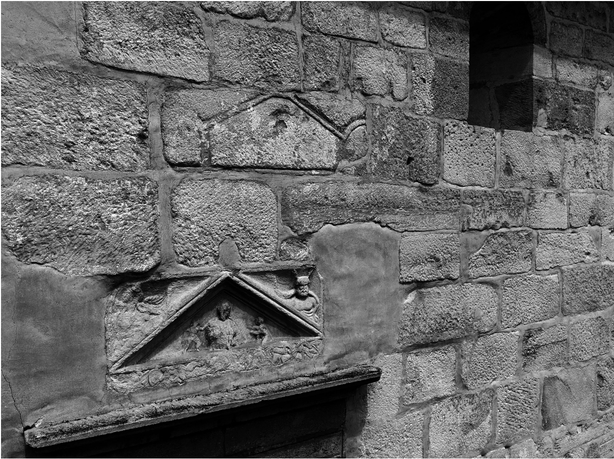
Figure 3. Marble spolia reused as building blocks in the south wall of the Romanesque church of St Michael in Črešnjevec
