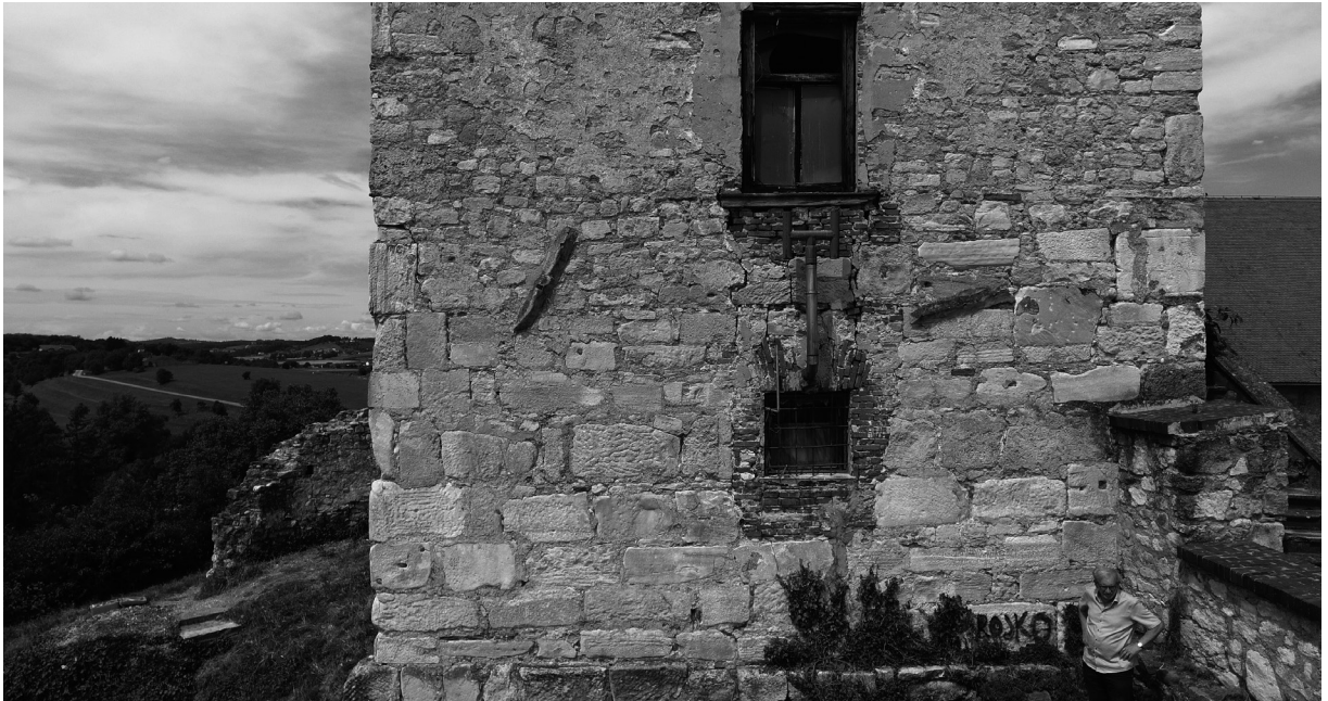
Figure 1. Marble spolia used in the construction of Ptuj Castle, here shown in the east façade of the west tower
