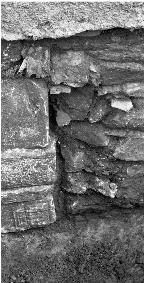
Figure 2. Foundations with marble spolia: Črešnjevec, church of St Michael, southwest corner of the first church (left), and Veliko Tinje, church of Sts Peter and Paul, northwest corner (right)
