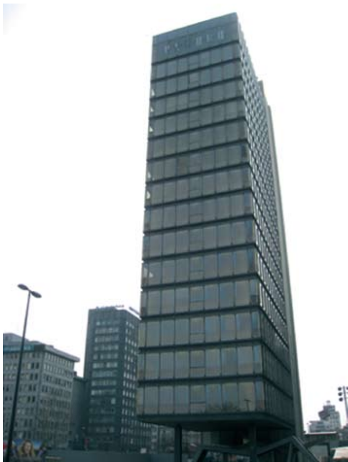
Slika 7: Milan Mihelič: jeklena konstrukcija nadstropij stolpnice S2 v Ljubljani. Figure 7: Milan Mihelič: Steel structure of the S2 high-rise in Ljubljana.
