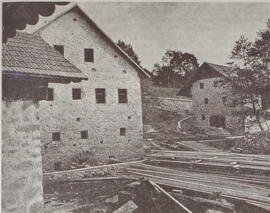
Trubar's Mill undergoing restoration (photo by Janez Zrnc)
