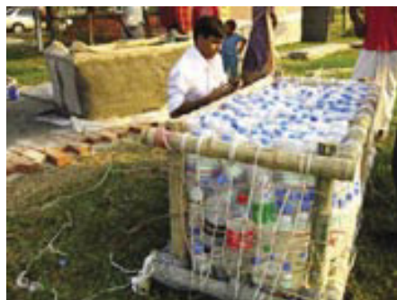
Slika 2 • Blooming Bamboo Home (Vietnam); plovno telo iz plastenk in bambusa ter prototip LIFT House (Bangladeš) ((Davis, 2013), (English, 2009), (Prosun, 2011))
