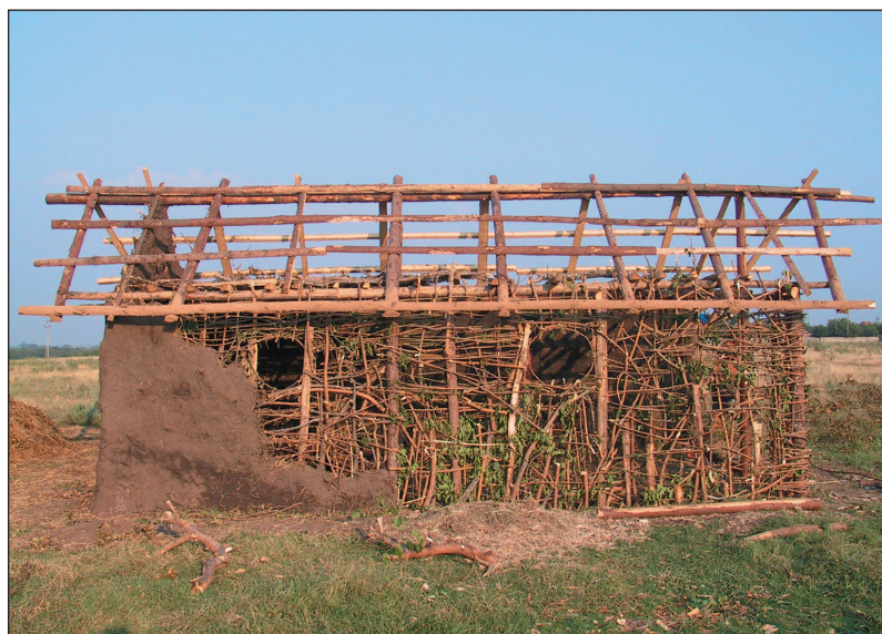
Fig. 5. The plaited structure of walls. Vadastra 2005.
