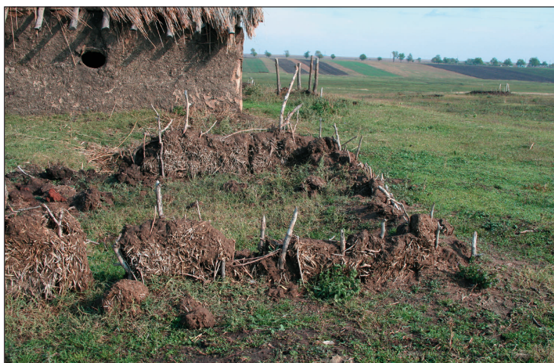
Fig. 8. The weathered walls of a wattle and daub house built in 2004. Vadastra 2007.
