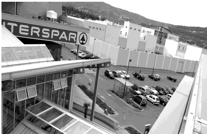
Figure 2: Shopping mall in Koper shares its parking lot with the city prison (photo: Domen Grögl).
