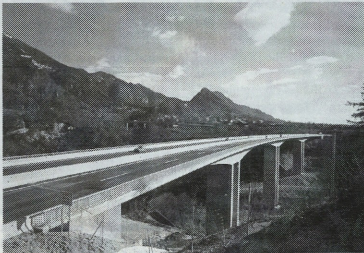
Viadukt Moste - ponos Gradisa
