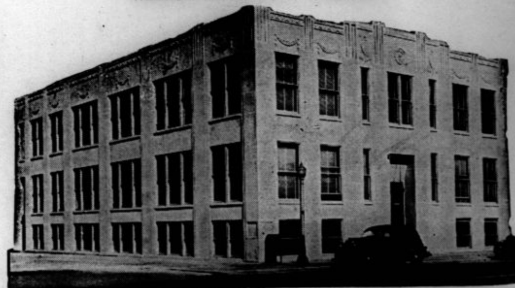
Photo shows the new K. S. K. J. Home Office Building. Entire foundation, floors and roof are Welsch Ready-Mix Concrete.
