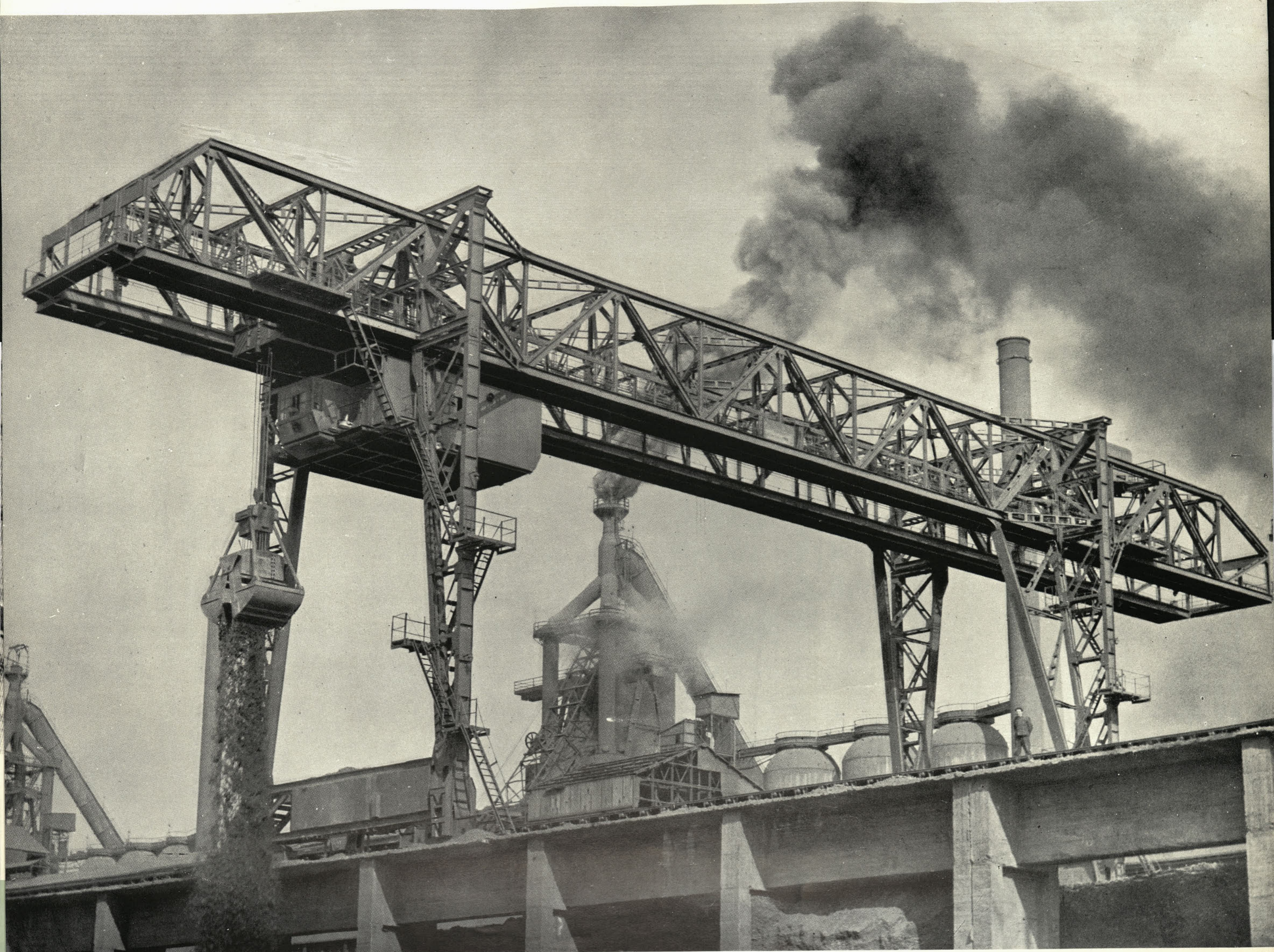
30-ton capacity crane with grab on ore yard of steelworks
