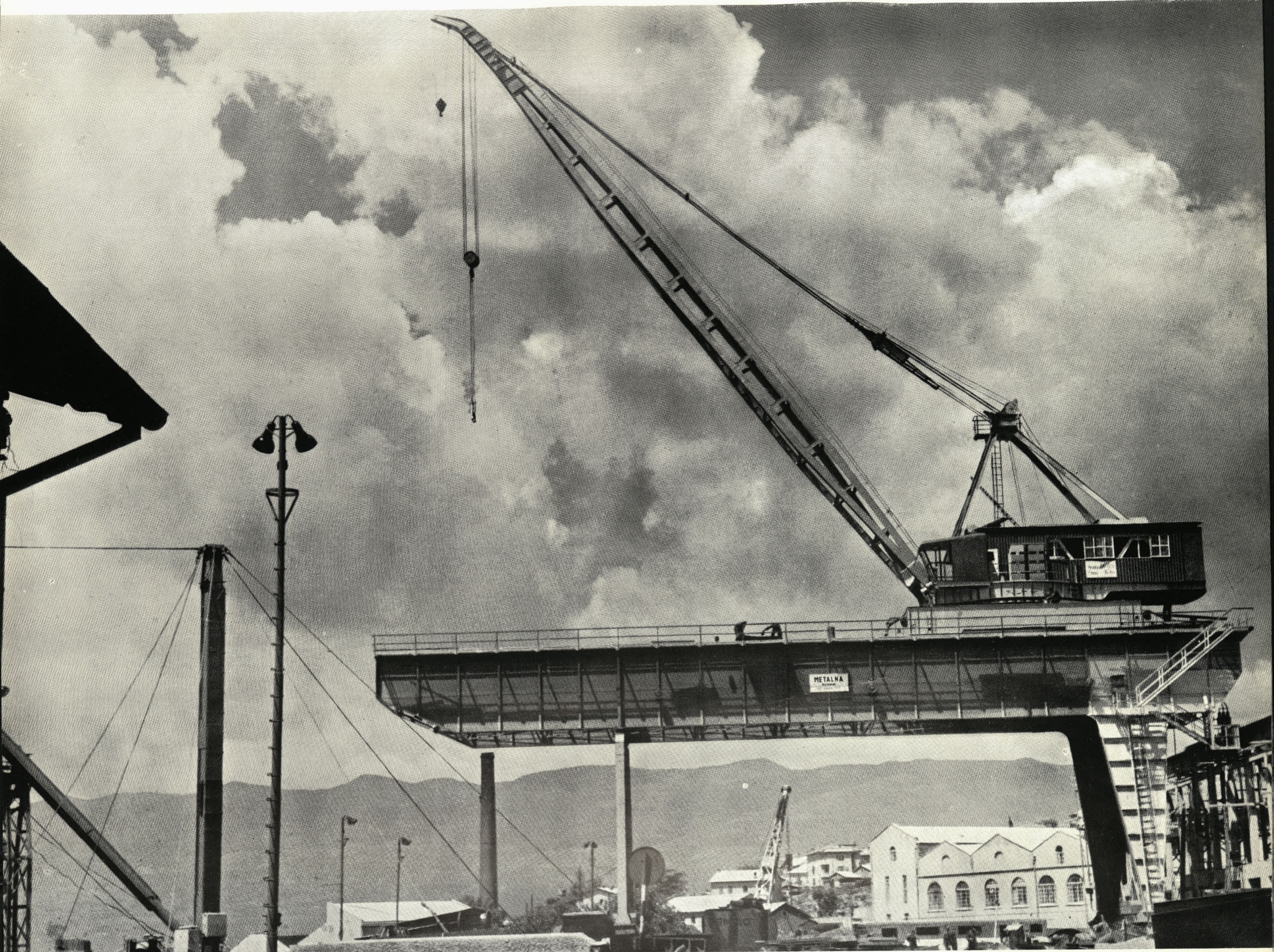
45/15-ton capacity shipyard crane
