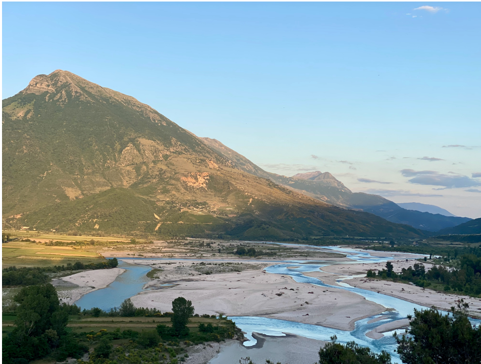
Figure 3: Middle catchment of the Vjosa River with complex flow patterns, predominantly branched and anastomosed streams
