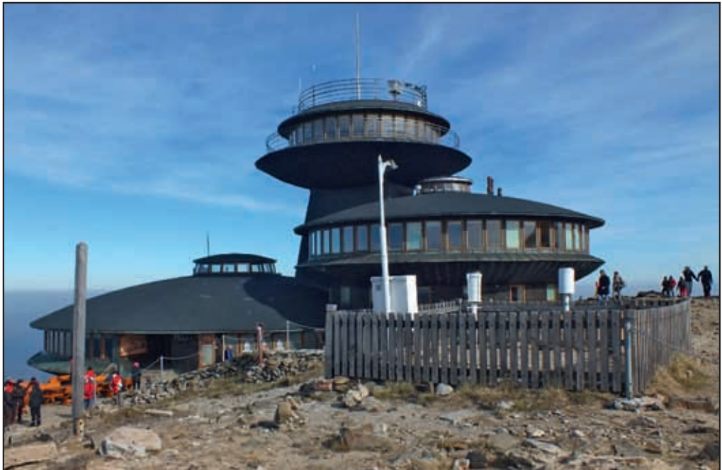
Figure 2: New IMGW-PIB observatory building at Mount Śnieżka.
