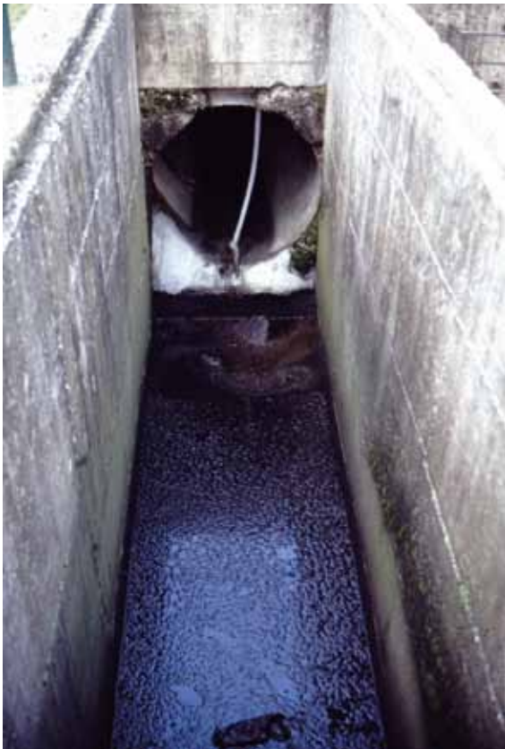
4 Dotočni jašek lovilnika olj A, kjer smo vzorčili dotočno vodo. Inflow shaft of the oil collector A where the samples were taken.
