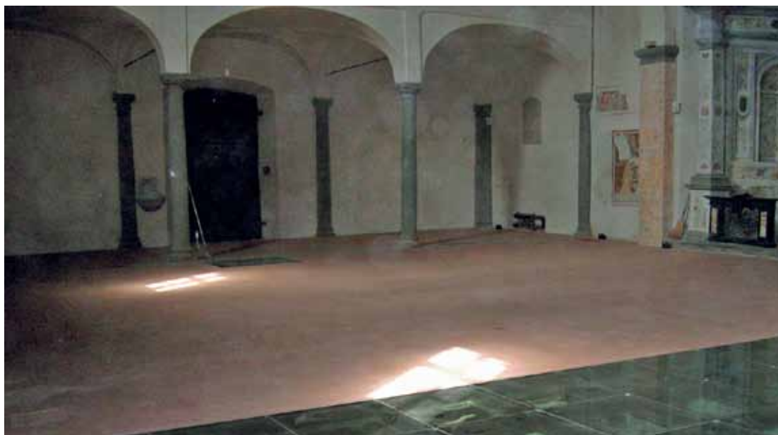
Fig. 19: Santa Maria del Lavello, the new pavement, partially opaque and partially realized with supporting glass tiles (Courtesy of G. Cruciani Fabozzi).
