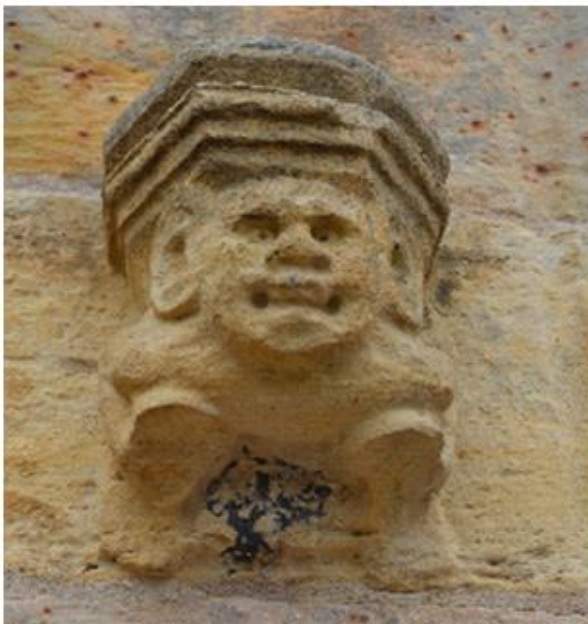
Damage made by acid rain on a statue in Scotland Photo: V. Kosmač, 2018
