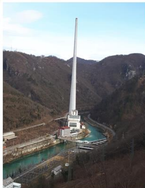
A power plant in Trbovlje in Slovenia. Photo: V. Kosmač, 2019
