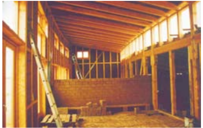
Slika 12: Naselje Landhof – predelne stene iz ilovnatih zidakov [Vir: zur Nieden in Ziegert, 2002:95]. The Landhof settlement – clay brick partition walls.
