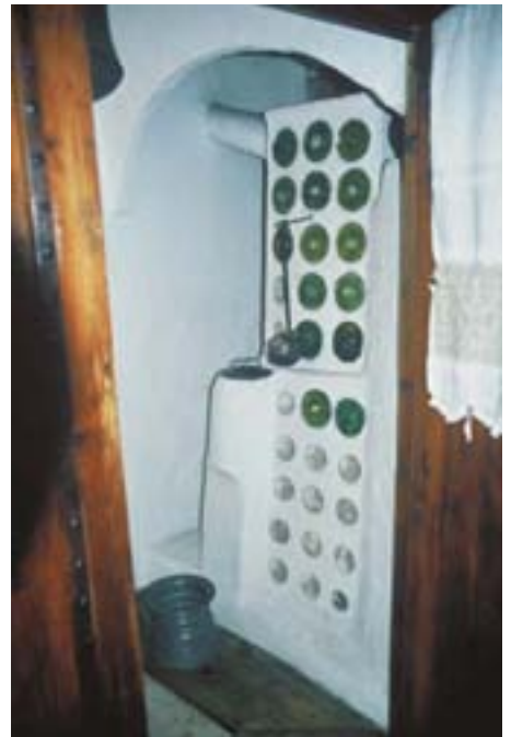
Slika 6: Skrb za osebno higieno – kopalnica za zidno omaro s pečjo (furuno) in ročno prho. Care for personal hygiene – bathroom behind the built-in cupboard with the furnace (furuna) and hand shower.
