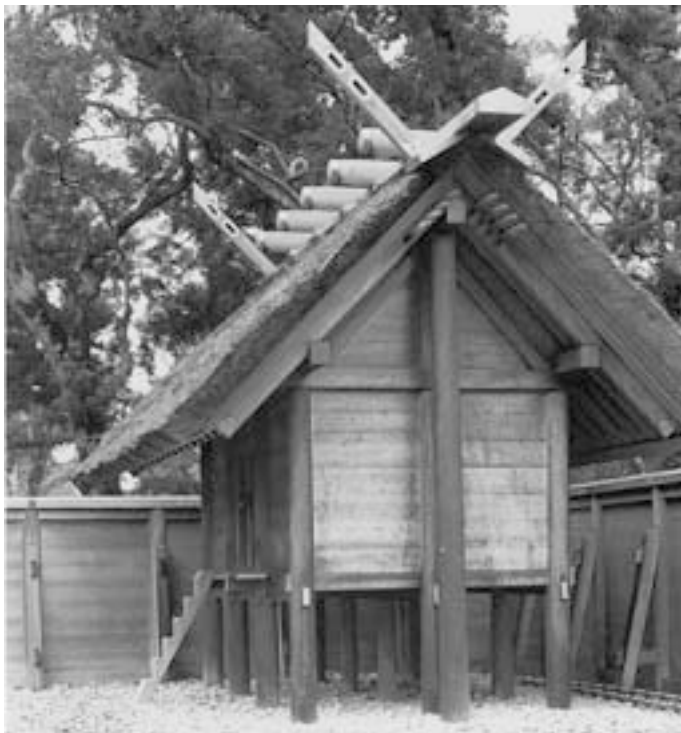
Slika 3: Odmik od terena in dodatni stebri, ki nosijo težo strehe. Distance from the ground and additional columns that bear the weight of the roof.
