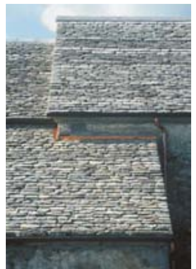
Slika 7: Obnovljena streha s kamnito kritino na cerkvi v Križu pri Sežani. Roof on the church in Križ, Sežana, renewed with stone roofing.
