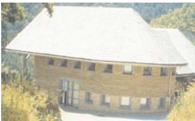
Slika 9: Ekološki center – južna fasada z velikim napuščem štiti ilovnate zidake pred meteorno vodo [Vir: zur Nieden in Ziegler, 2002:126]. Ecological centre – south facade with large overhanging that protects the clay bricks from rain water
