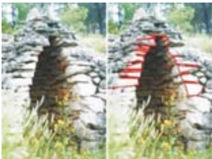
Slika 2: Prerez korbelinga v praksi: majhen trim kot zatočišče za enega človeka. Section of corbelling in practise: the small trim as a shelter for only one person.
