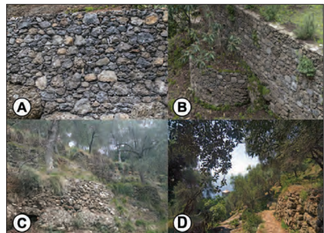
Figure 8: Dry-stone walls in conglomerate: (A) dry-stone walls in conglomerate mixed to limestone (B) olive grove (C), (D) San Fruttuoso’s environment and terraces Photo by: A. Girani.
