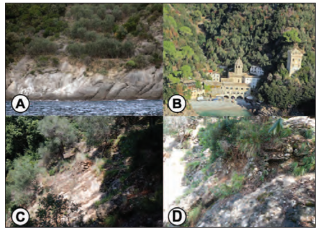
Figure 5: Terraces of olive groves close to the sea (A) San Fruttuoso Abbey, (B) incidents of collapse and other cases of geo-hydrological deterioration such as soil erosion and landslides in the wake of abandonment or poor maintenance of dry-stone walls, (C), (D) Photo by: A. Girani, F. Faccini.
