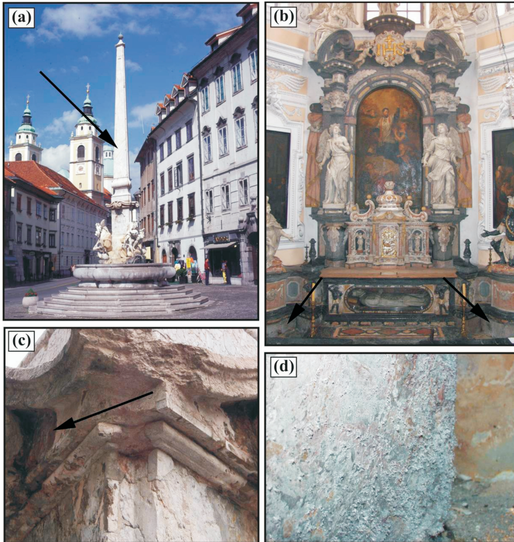
Figure 1. Selected monuments and weathering forms of Lesno Brdo limestone. (a) Fountain of the Three Carniolian Rivers - the obelisk is made of Lesno Brdo limestone, and the statues of Carrara marble. (b) Side altar of the Church of St. James. Some of the stone elements of the lower parts are made of Lesno Brdo limestone. (c) The black crusts are compact aggregates of salt minerals, occurring on the surface on sheltered areas. The Figure shows a detail of the obelisk of the Fountain. (d) Fluffy efflorescence, appearing as very loosely coherent aggregates of acicular and long hair-like crystals. The Figure shows a detail of the lower part of the altar. The width of the image is about 10 cm.
