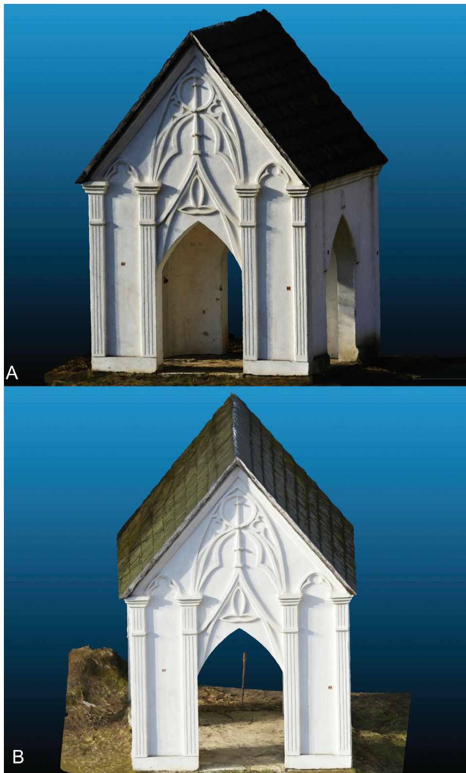
Figure 60. Žehra, Hodkovce (Slovakia). Neo-Gothic park architecture (19 th century), exterior. lBM (325 photos 24Mpx). Isometric views of the textured 3D model. A: visualisation with normals, B: visualisation without normals.
