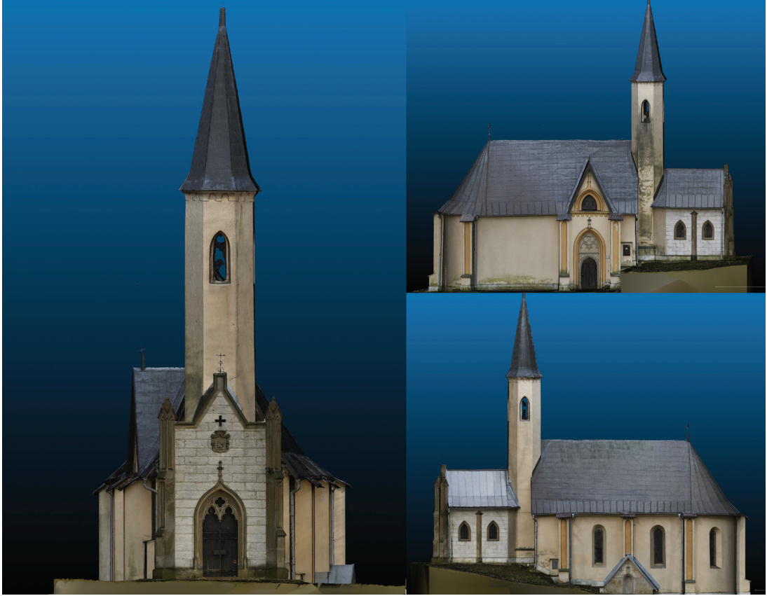
Figure 56. Žehra, Hodkovce (Slovakia). Neo-Gothic church (19 th century), exterior. lBM in combination with TLS. Ortho-views of the facades.
