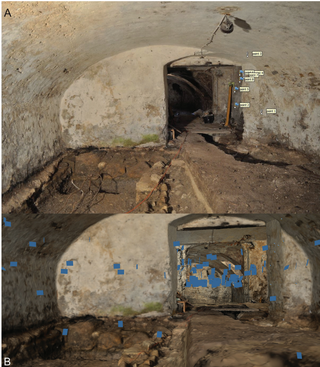
Figure 66. Rajec (Slovakia). Burgess house (16 th century), cellar. lbM (217 photos 12Mpx). A: example of raw photos with markers indicating control points, B: distribution of cameras.
