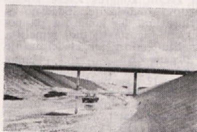
Most v km 2+376
