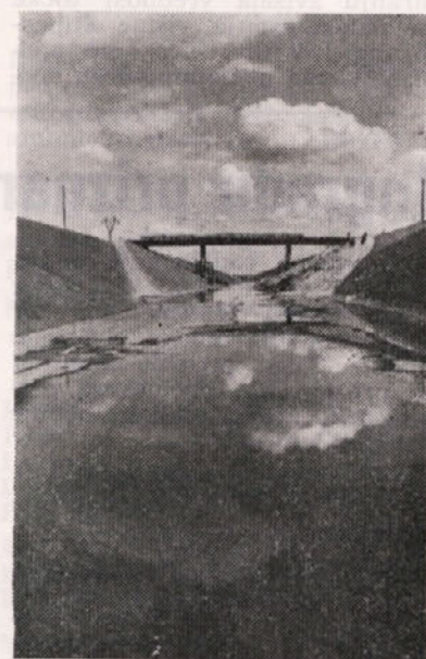
Most v km 4+382
