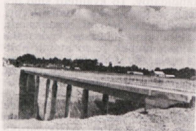
Most v km 8+738
