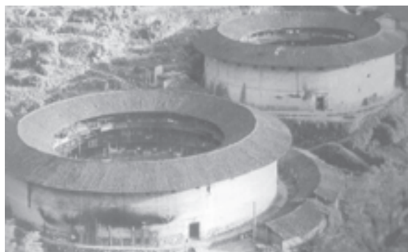
Slika 4: Večstanovanjske zgradbe manjšinskega plemena Hakkas iz butane ilovice v kitajski provinci Yoding. Multi-apartment buildings of the minority tribe Hakkas in the Chinese province Yoding made from compacted clay.
