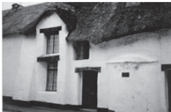
Slika 8: Najbolj znana angleška zgradba iz ilovice, pomešane s slamo v Devonu iz leta 1539. The best known English building made from clay mixed with straw, built in Devon in 1539.
