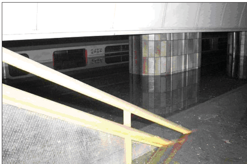
Figure 11. Submerged metro train in Florenc Station (after some of the water had been pumped out).
