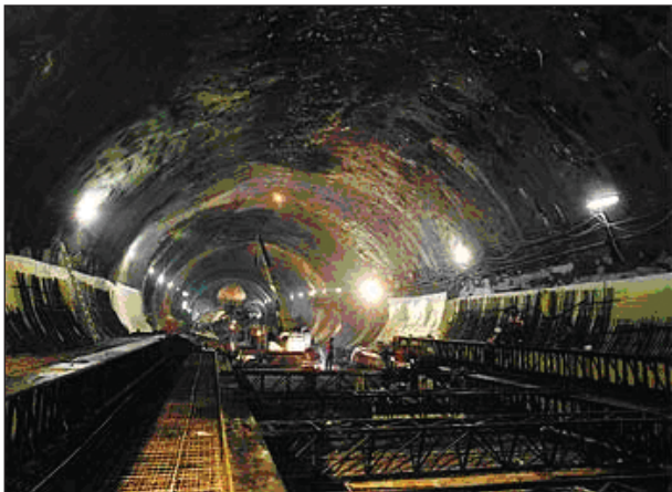
Figure 8. The building of the Kobylisy station.
