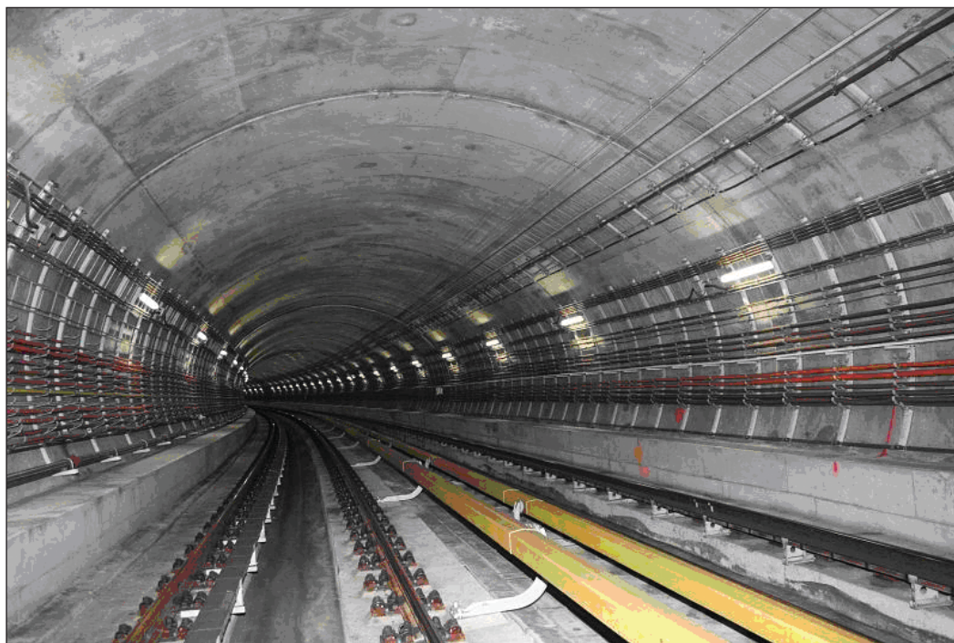
Figure 3. Double-track metro tunnel on line C.
