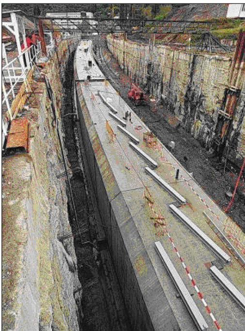
Figure 9. Immersed tunnel – the concrete tube still in the dry dock.
