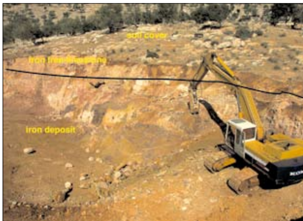
Fig. 2 a,b: Views of the current pit mine that exposes the iron ore body underneath a fragmented limestone layer. The pictures were taken in November 2005.
