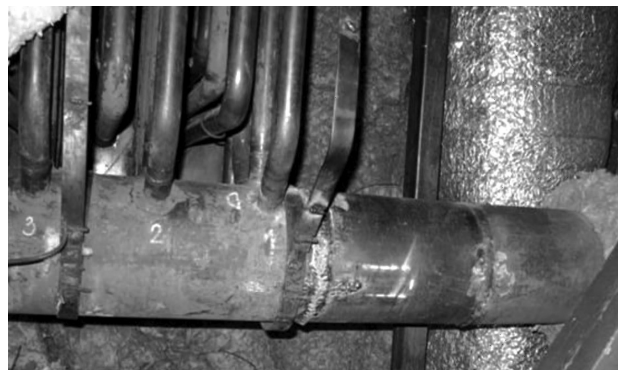
Figure 2: Support of the superheater collector Slika 2: Del zbiralnika v pregrevalniku
