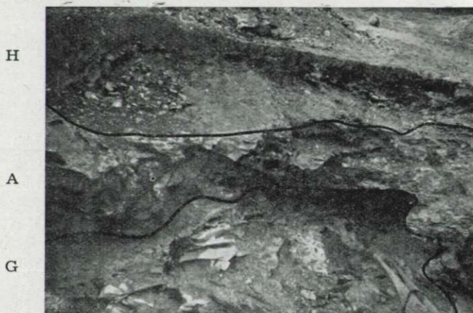
H humus in zdrobljen apnec A bituminozni apnec G montmorillonitna glina Humus and crushed limestone Bituminous limestone Montmorillonite clay
