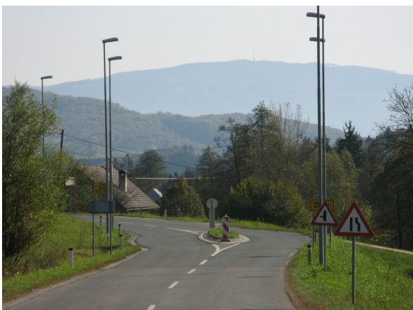
Fotografija 3: Ureditev za umirjanje prometa Photo 3: Road adapted to the reduced speed
