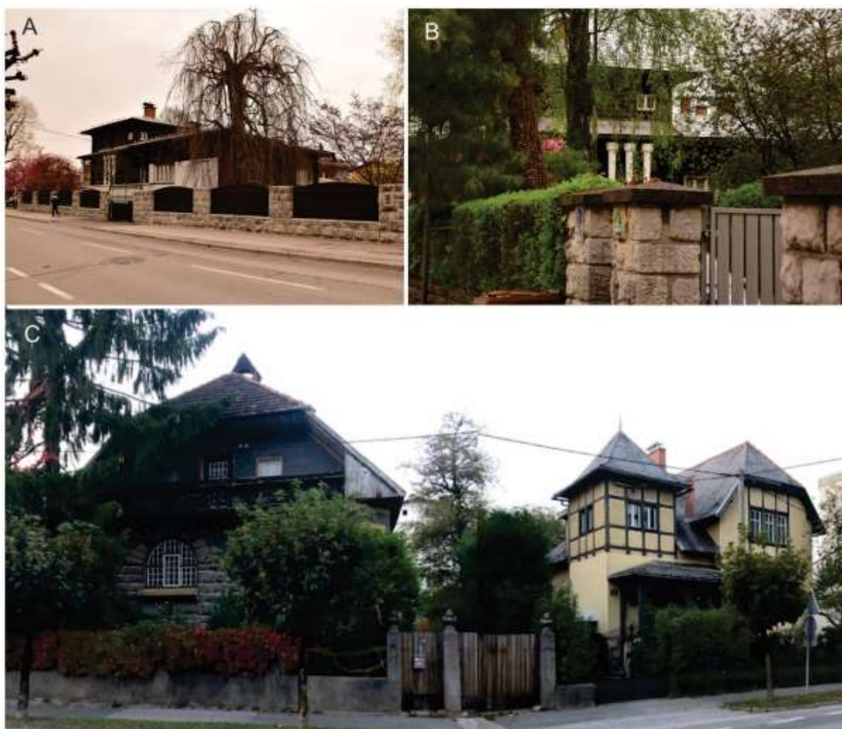
Figure 6. Villas in Mirje district (Jamova ulica) (Nos. 3, 6 and 7 in Figure 2 ).
