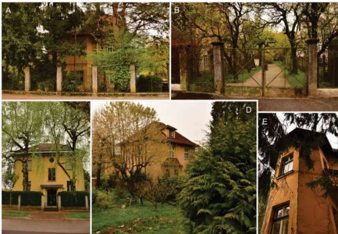
Figure 5. Villas in Mirje district. A,B,D,E: Teslova ulica (A,B: No.4, D: No.5, E: No.2 in Figure 2).
