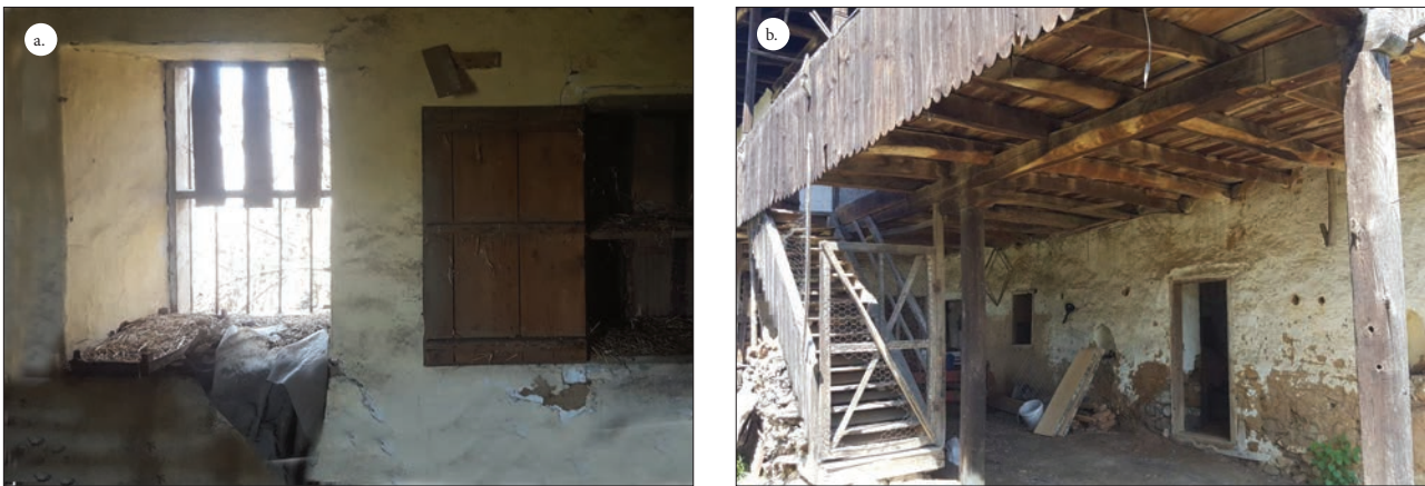
Figure 12: A traditional house in Janchishte, Tetovo: a) the wide parapet of a window; b) the floor with wooden planks and beams above the hajat (Photo: Aurora Saidi).
