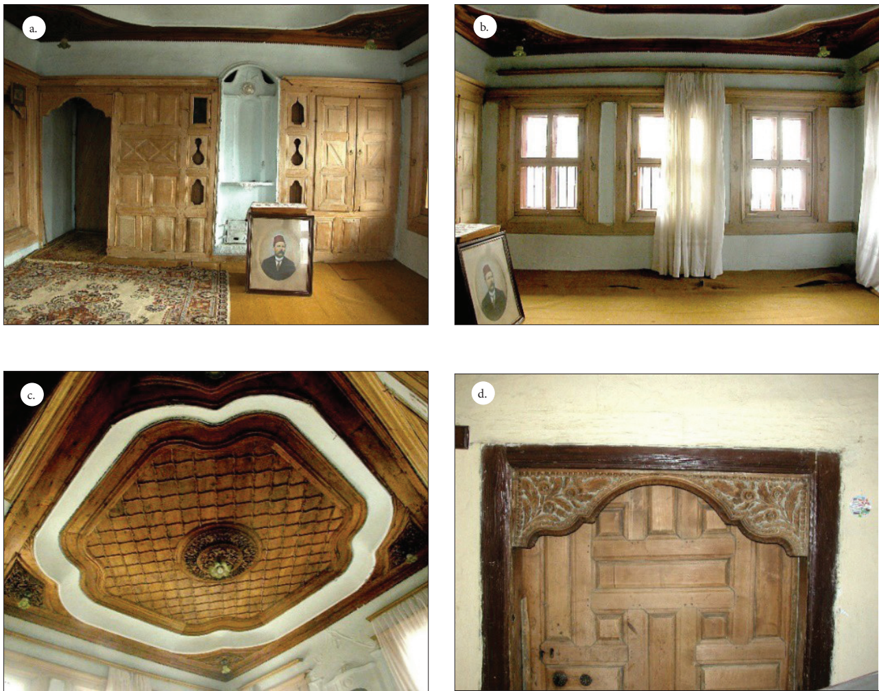
Figure 11: An illustration of the interior of a traditional house in Tetovo. The house of Mehmet Palloshi, Tetovo: a) musandra – in-wall closets and cupboards; b) windows; c) decorated ceiling; d) decorated doors (retrieved from Kiprianovski & Trajkoska, 2007).
