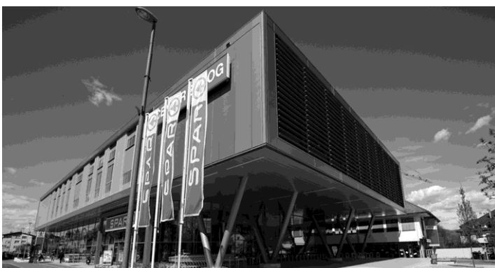
Figure 10: The new commercial building in Zalog in oversized format (photo: Domen Grögl).
