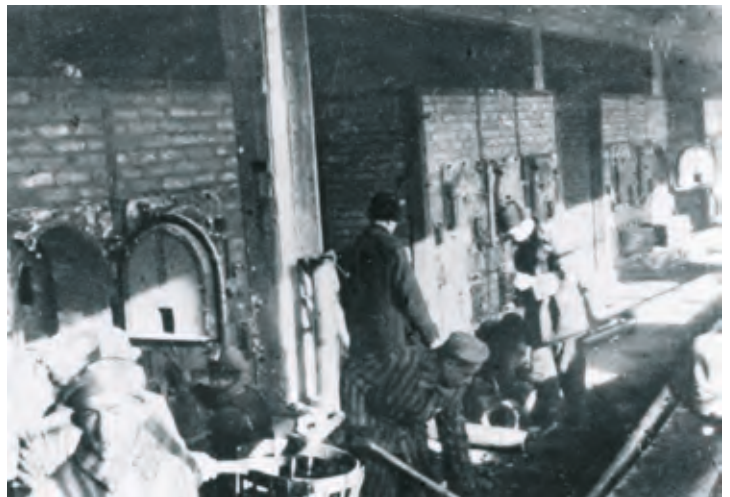
Forced laborers building the crematorium in Auschwitz (photo credit: Yad Vashem, Jerusalem)
