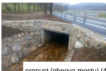
prepust (obnova mostu) (4)
