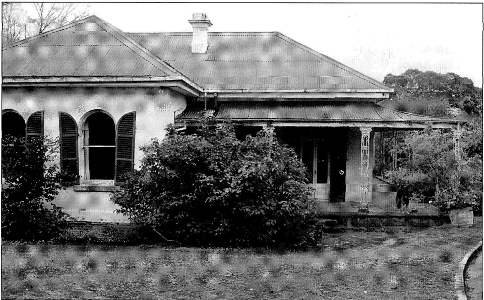
Fig. 4: Part of the south side of the main house at Varroville. The cast iron veranda columns on the right were added in 1859, but at least part of the house was built in the 1820s. Photograph by Ian Leister 17 Sept. 1995.
